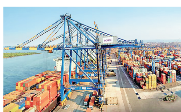
The company plans to develop a 25-metre-deep port that can accommodate Panamax vessels. Representational
